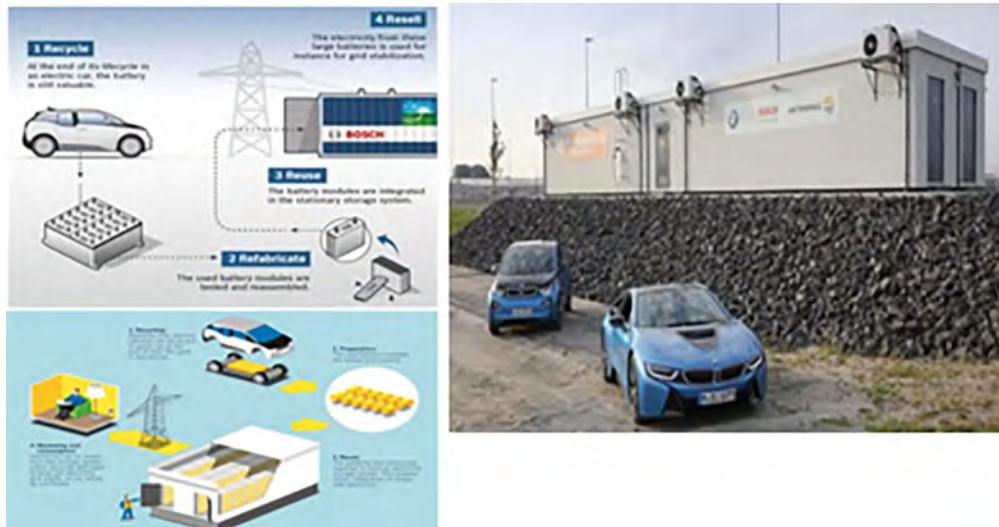
Figure 4.6: BMW–Bosch Second-Life Electric Vehicle Battery Demonstration Project
