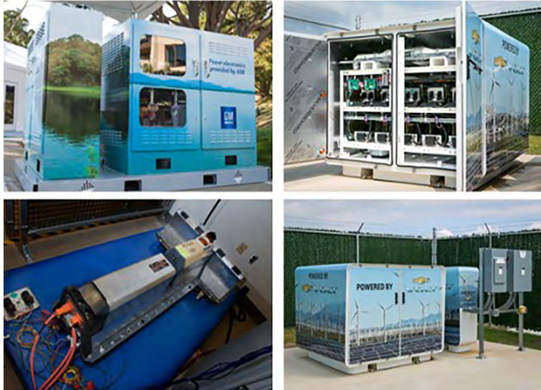
Figure 4.4: GM-ABB Second-Life Electric Vehicle Battery Applications
